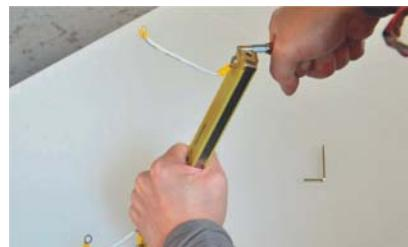
7. Fasten the heating wire by Allen key, then cut the remaining heating wire by the special tool.
